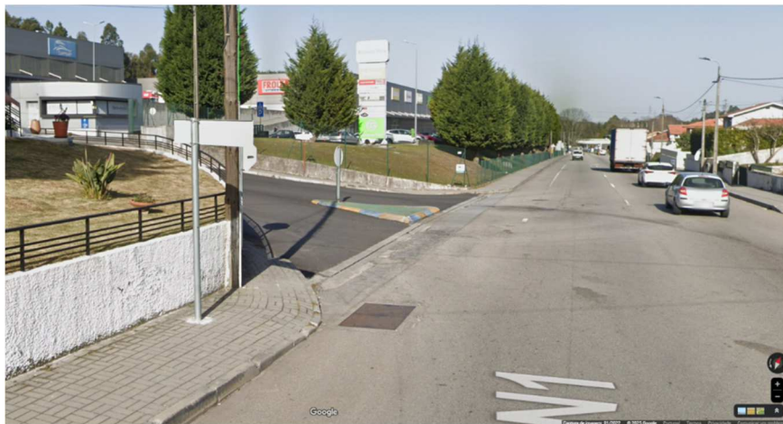
figura 7. Estrada N1 [Google Street View, 2025]
